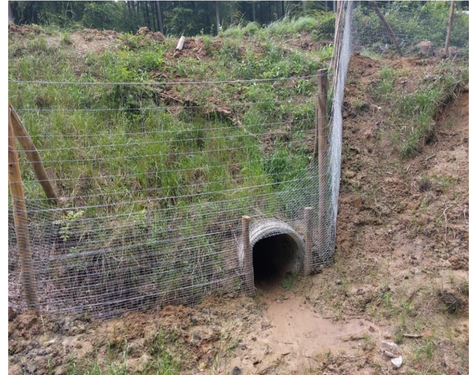
Newly pressed ecotunnels
